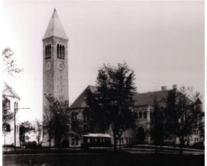
McGraw Tower with trolley.
